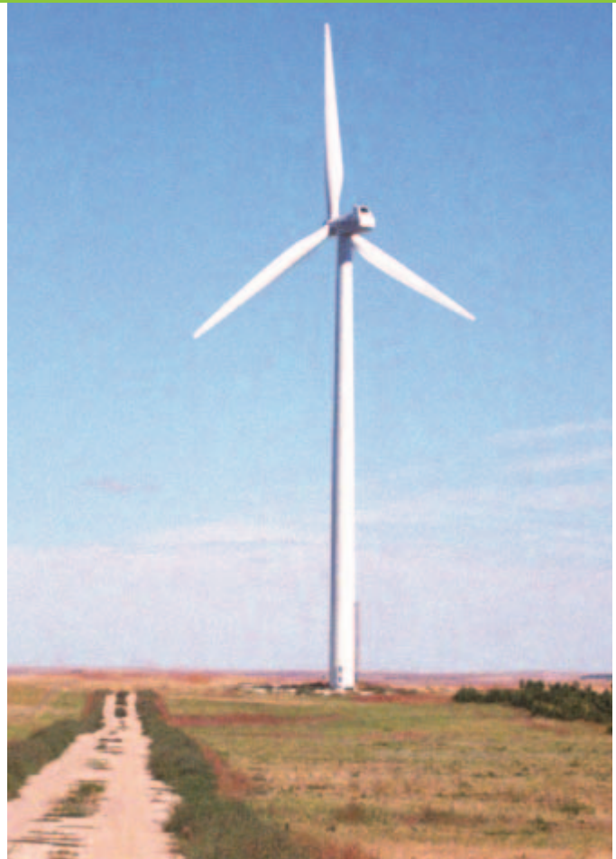
In May 2003, the Rosebud Sioux tribe dedicated the first Native American utility-scale wind turbine on their reservation in South Dakota.
